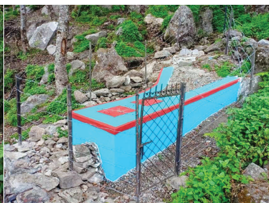
Construction of intake in the community
