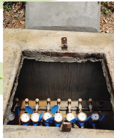
WATER METER AND DISTRIBUTION POINT
